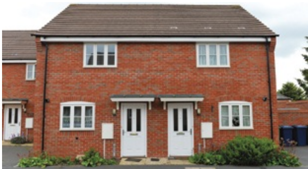
semi-detached house la casa pareada
