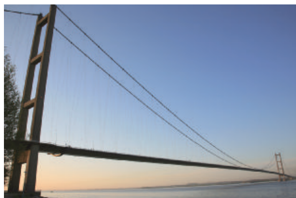
The suspension cables on this bridge are also parabolas.
